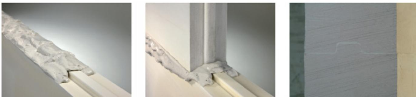
Thoroughly applied adhesive ensures stability, sound insulation and fire resistant properties of the whole structure of gypsum boards.
