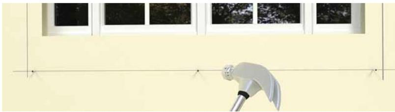
In order to ensure the straight line of alignment of the profiles, their precise positioning should be carried out with a leveler or by using a powder drawing instrument with twine. With their help the position of the profiles on the facade is marked. On the bottom line, over 1 m are
