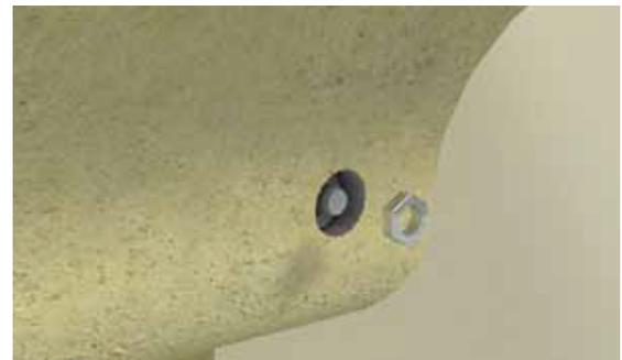
The hole is cleaned (blown) from the remaining from the drilling and filled (only the hole in the base) with chemical dowel. The dowel is shortened to the required length (so that the end remains inside the profile without pointing out of it) and it is hammered with a hammer firmly into the base through a hole in the profile. The area around the dowel in the profile is filled with TERMOFLEX® PU CONTACT. The spit and nut are rolled carefully by hand. After 24 hours their final tightening is done.
