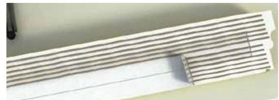
Using a notched trowel (4x4 mm), TEHNOCLAY® ADHESIVE FOR DECORATIVE PROFILE FROM EPS is applied first on the base in the marked area. Small unevenness can be leveled with more adhesive. After that the adhesive is applied on the entire surface, on the back of the profile, which with slight, side movements is pressed against the wall in order to optimize the adhesion. The indicative consumption of the adhesive is about 8 kg/m<sup>2</sup>.
