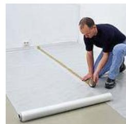
The noise and thermal underfloor insulation should be applied in rows in the same direction which will be chosen for the application of the laminate/ parquet. A gap around 2 mm should be left between the separate boards. Avoid placing the overlaps of the underfloor insulation and the laminate/ parquet at the same spot. Between the underfloor insulation and walls, columns, thresholds, etc. Leave 1cm gap to the walls, door-sills, columns, etc. to cover the temperature extensions.
